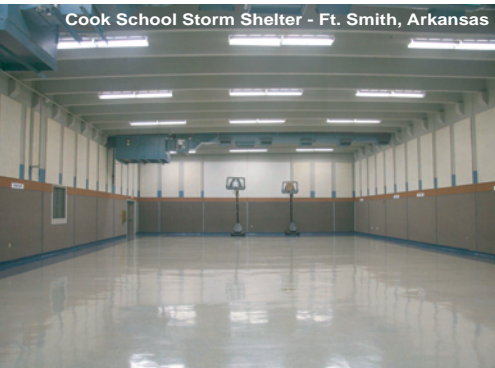
Cook School Storm Shelter - Ft. Smith, Arkansas
