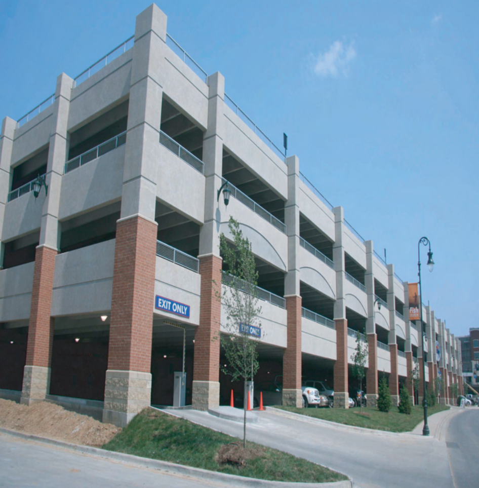
Branson Landing Parking Garage - Branson, Missouri
